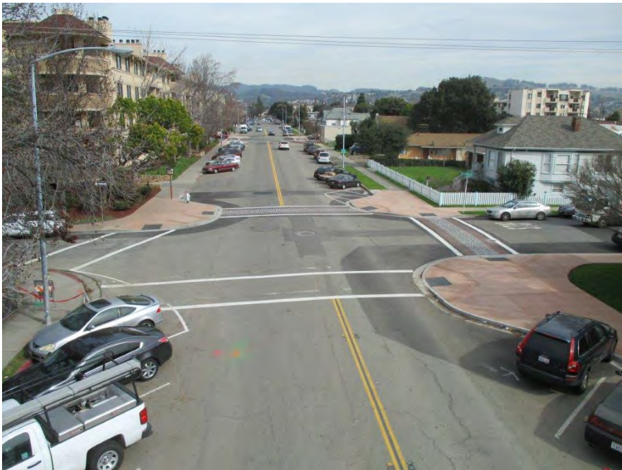
The West Juana Street Pedestrian Improvement project was completed in FY2016.
