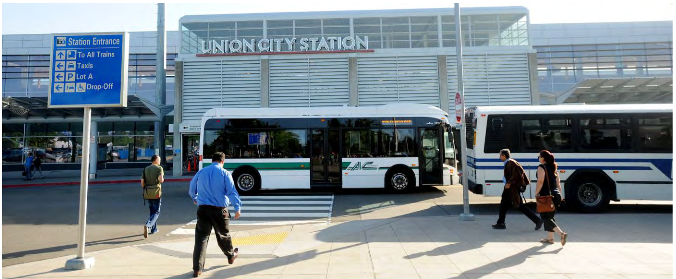
Union City Intermodal Station
