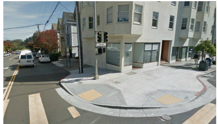
Bulb-out with crosswalk dual ramps Source: SF Streets Blog
