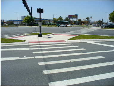
Continental marked crosswalk
