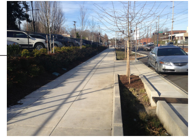
Stormwater planter between sidewalk and street parking
