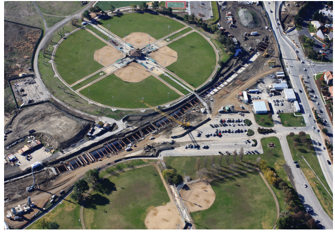
Construction on BART Warm Springs Extension
