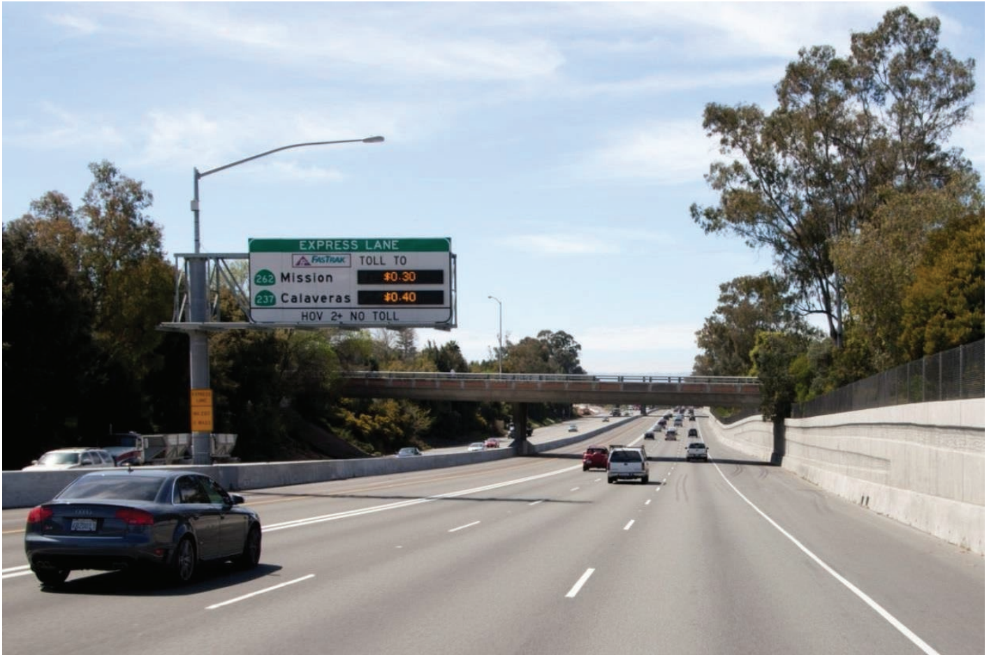
Existing Southbound I-680 Express Lane Signage
